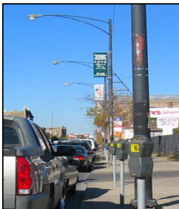
Existing light poles on Milwaukee Avenue are mostly on the east side of the street.
