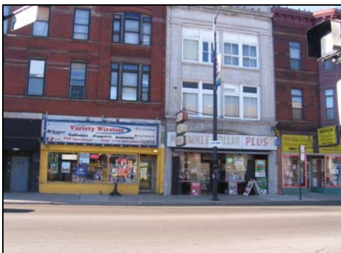
Several buildings would benefit from rehabilitation and renovation.
